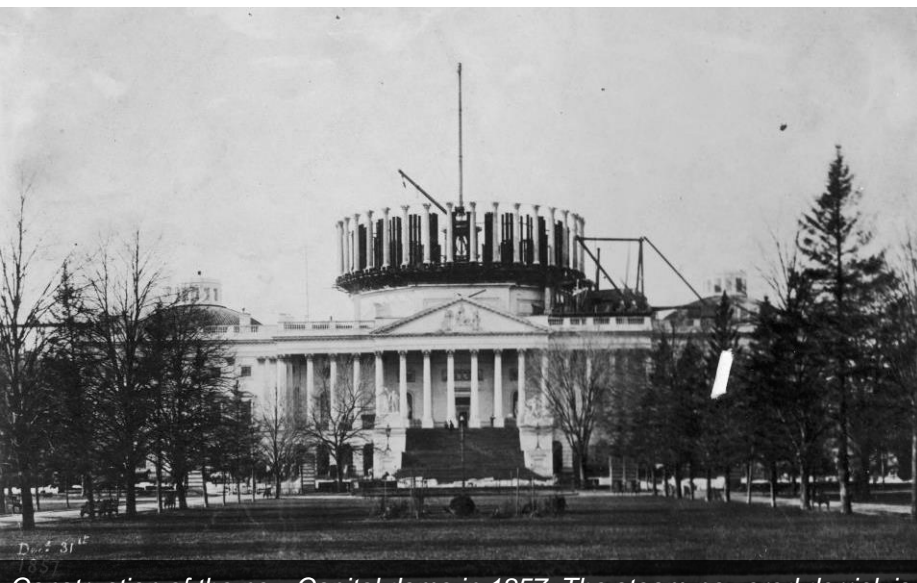
Construction of the new Capitol dome in 1857. The steam-powered derrick is visible above the building. (Architect of the Capitol)
